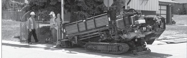
Ting is currently in the 1st Phase of fiber optic install in Walnut Hills, making holes for access points for conduit and junction boxes. Holes are produced using vacuum extraction thereby minimizing damage in the right of way. (Photos - Jesse Alcorta)
