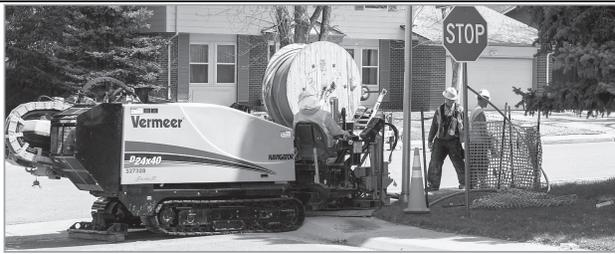
Construction continues utilizing horizontal drilling equipment for drilling in the right of way for conduit to be pulled through from block to block. Conduit lays approximately two feet below the surface to minimize the impact on other services.
