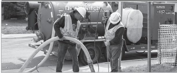
Ting is currently in the 1st Phase of fiber optic install in Walnut Hills, making holes for access points for conduit and junction boxes. Holes are produced using vacuum extraction thereby minimizing damage in the right of way. (Photos - Jesse Alcorta)
